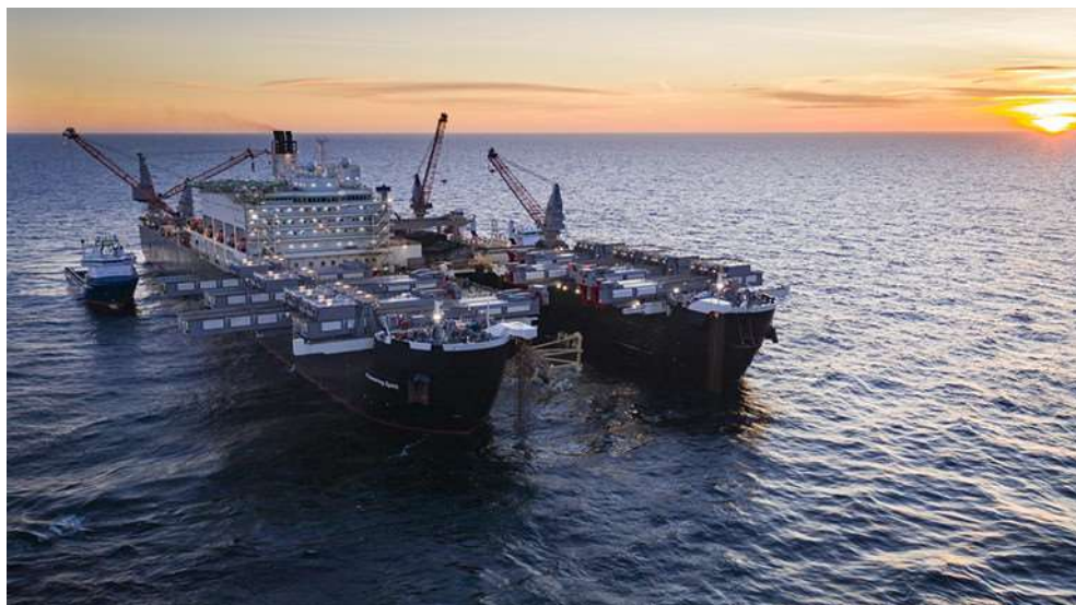
Offshore work being carried out for Nord Stream 2. (Gazprom)
